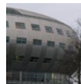
HOLLAND Hot water pumping across district network
