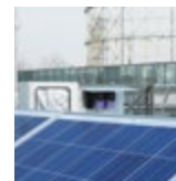
ITALY Cooling loop flow & temperature control
