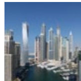
DUBAI Saving energy in air conditioning systems
